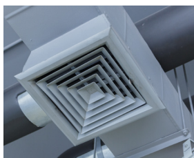
Ventilation duct monitoring
